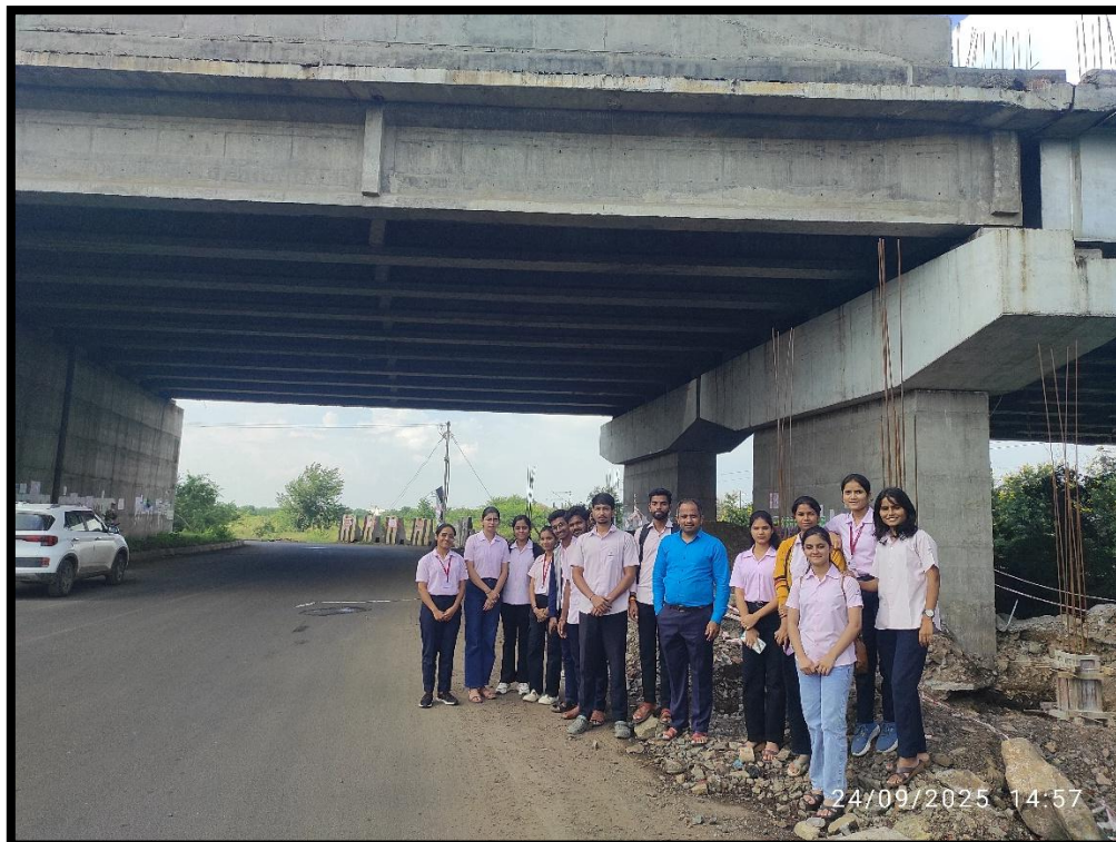
Fig. 4: at Bridge site near Airport and Railway track junction on palkhi mahamarg
